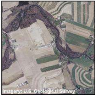
SITE 1 - Tenupy Bridge
